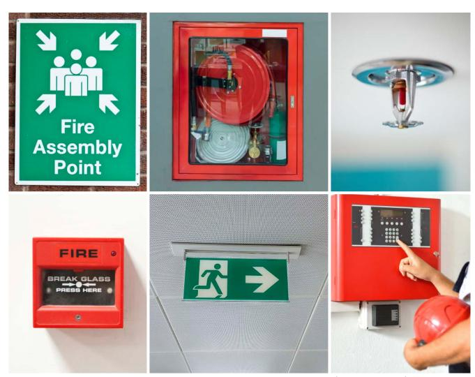
Figure 3.1 Examples of Fire and Life Safety Equipment and Signage (clockwise from top left): Assembly Point Sign, Fire Extinguisher inside Hose Reel Cabinet, Automatic Fire Sprinkler, Fire Alarm Control Panel, Exit Sign, Fire Alarm Call Point
