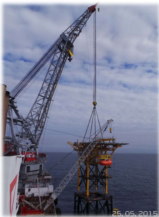
Figure 3-8 Lifting of Topside (example from erecting).
