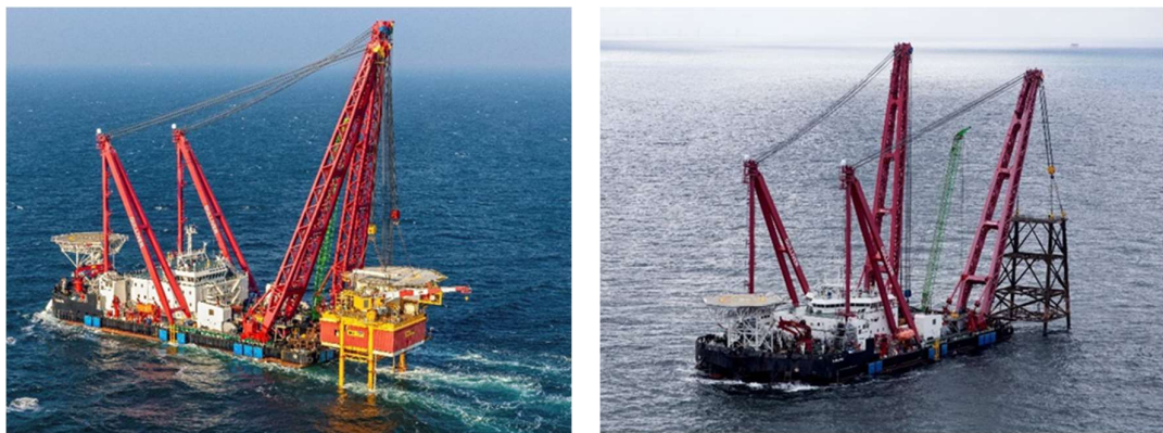
Figure 6-17 Examples on transport of Topside and Jacket in crane hook.
