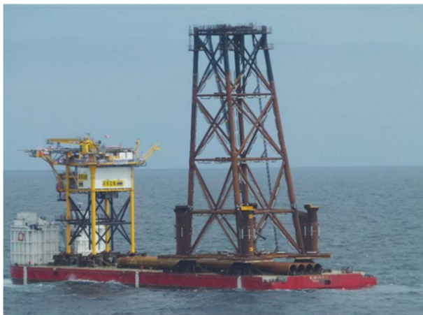
Figure 6-18 Example of transport on barge.
