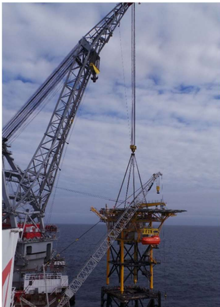
Figure 6-13 Lifting of Topside (example from erecting).
